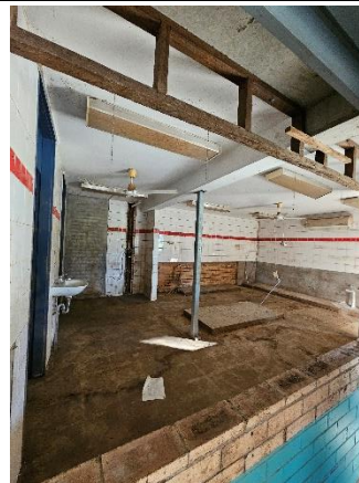
Photograph 6: Ground floor canteen area B00E
