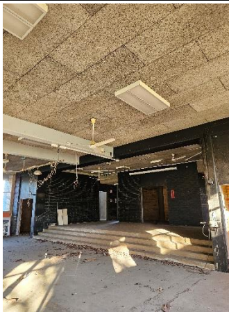
Photograph 5: Ground floor hall B00A
