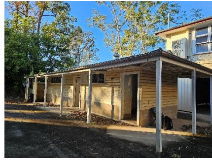
Photograph 8: B00G toilet block
