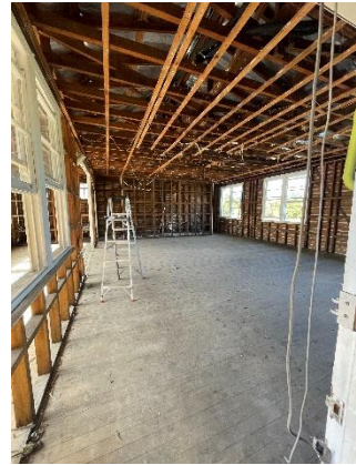
Photograph 4: Internal areas of B00H
