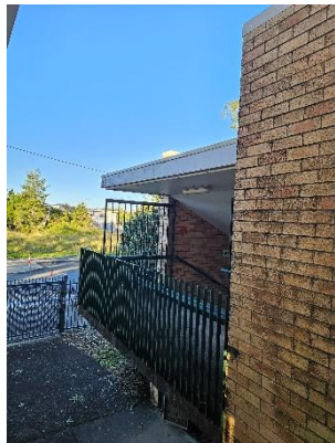
Photograph 9: B00I stairway and movement areas.
