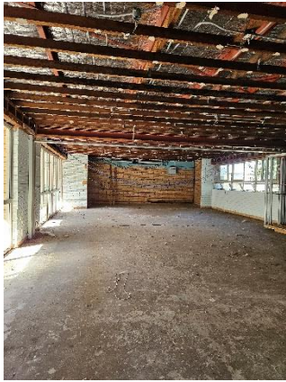
Photograph 7: Internal classroom area B00D
