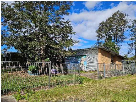
Photograph 17: Building B00J - preschool
