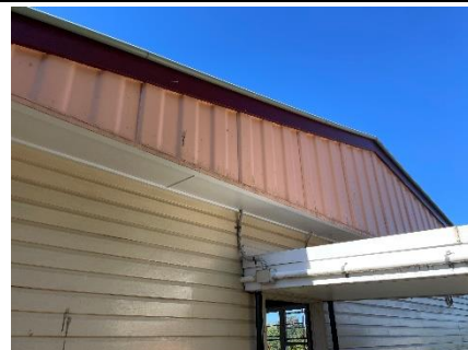
Photograph 24: Roof gable ends and eaves to building B00H (Asbestos detected in roof gable end and eave lining)
