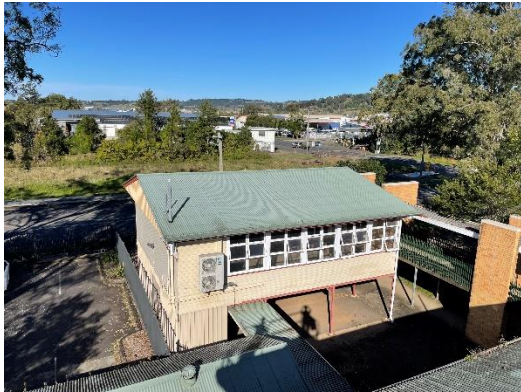
Photograph 3: Building B00H looking south
